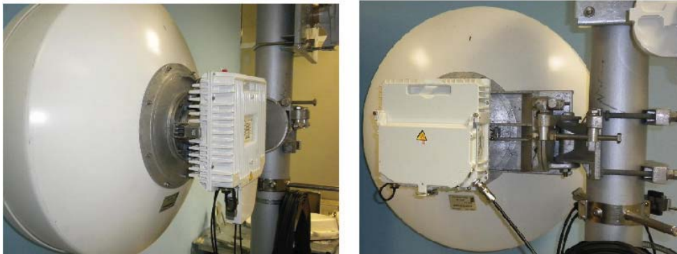
Figure 13. MPT-HC (11-38 GHz on the left side; 6 GHz on the right side)
