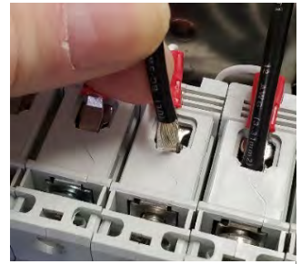
Figure 8 Connecting the load
