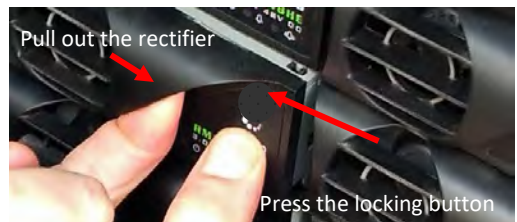
Figure 15: Removing a Rectifier
